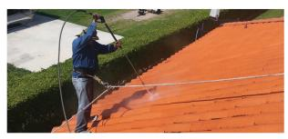
**SURFACE PREPARATION:** All surfaces must be clean, dry, and sound; free from loose and peeling paint, dirt, wax, grease, oil, efflorescence, curing agents, mildew, and other detrimental foreign matter that will adversely affect adhesion and product performance.
